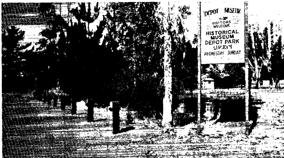
Trail access to Depot Park, 1985.
