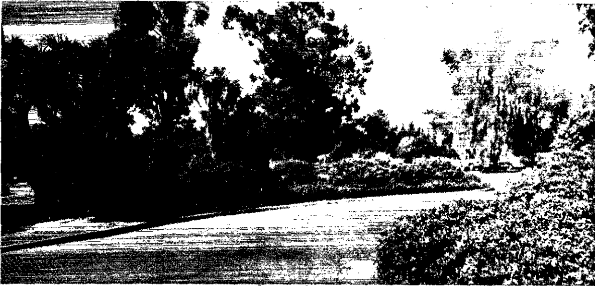
Current entrance road and landscaping, 1985.
